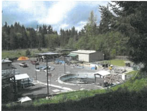
Granite Falls Wastewater Facility
